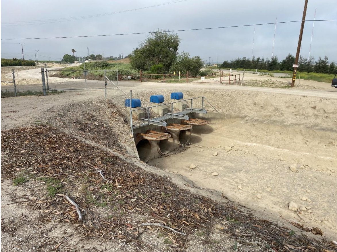
Figure 1: Looking West at Existing Channel and Road Crossing
