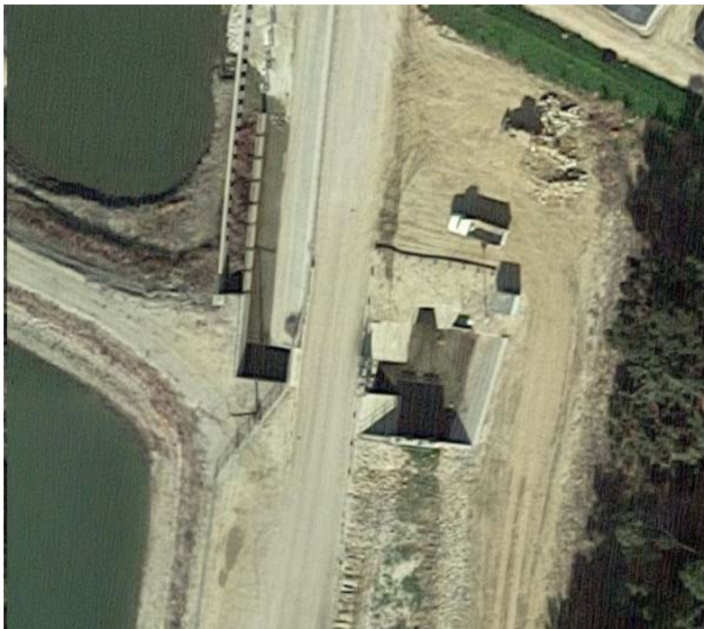
Figure 13 Inlet to the existing desilting basin
