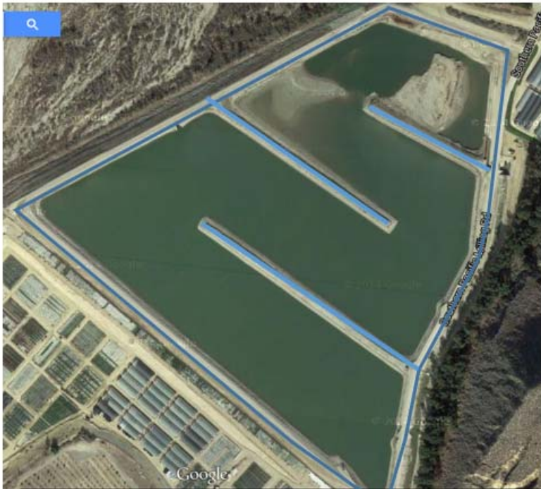
Figure 12 Aerial view of the existing desilting basin
