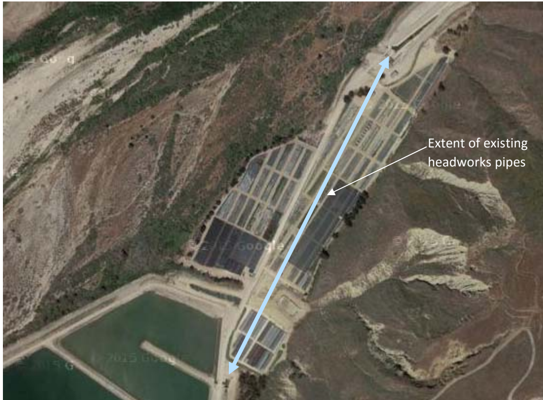
Figure 12. Aerial view of the headworks pipes are
