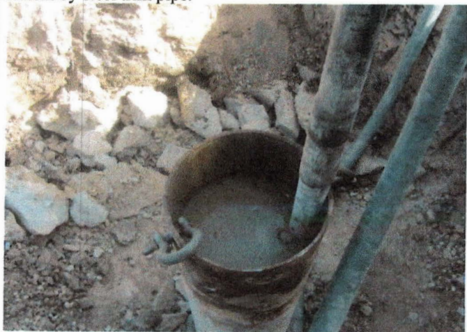
Neat cement to surface inside casing.
