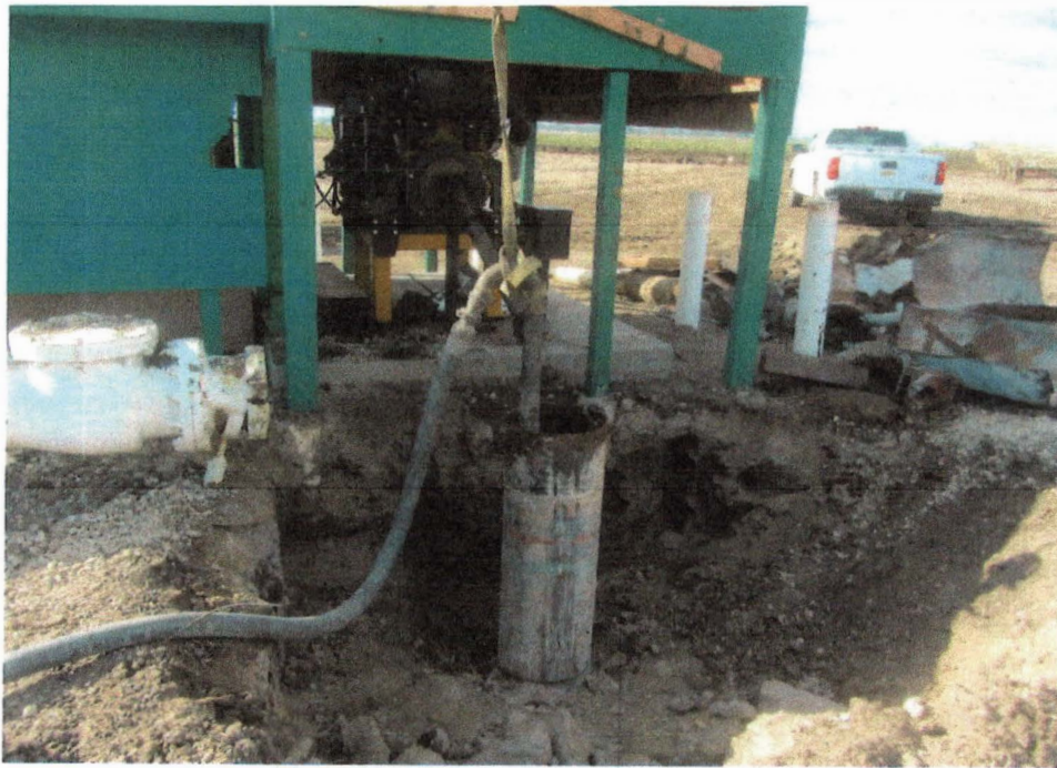
Placement of neat cement by steel trim pipe.
