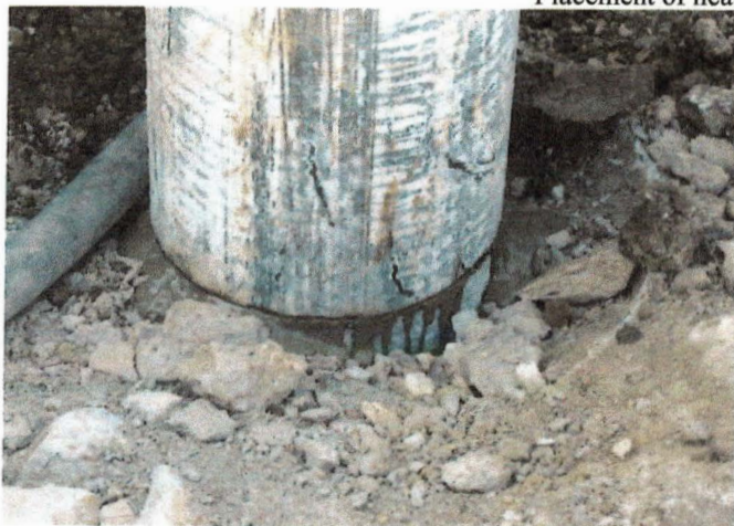
Neat cement seeping from casing where it is cut 5 ft down.
